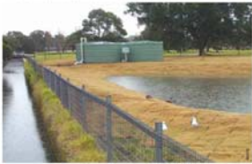
Barnwell Park Golf Course - stormwater channel, retention basins and storage tanks - Australia
