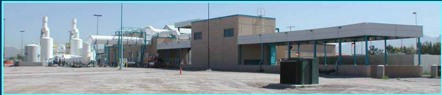
Ina Road WRF Headworks
